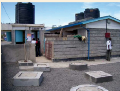
New Public Sanitation Facility
