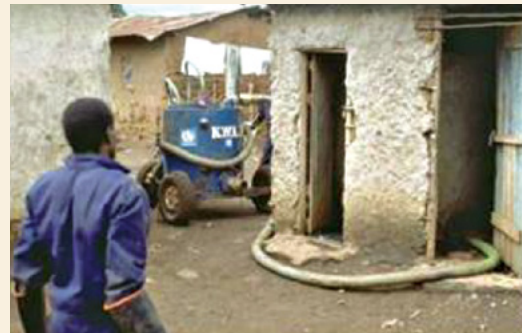
Vacutug: improved technology for mechanical pit emptying
