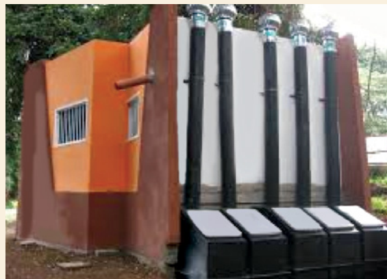
Ikotoilet Urine Collection System, City Park, Nairobi
