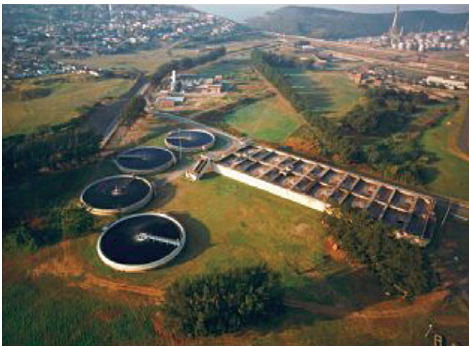
Durban Wastewater Recycling Plant
