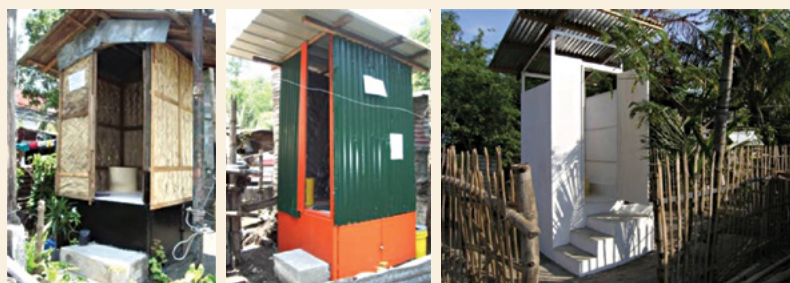
Construction of UDDTs in various materials
