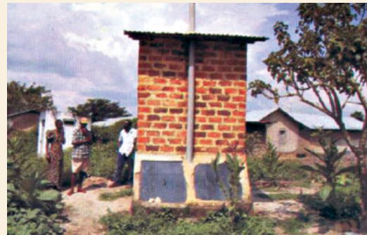
New Ecosan toilet: no emptying service in place
