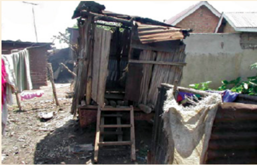
Poor quality of toilets
