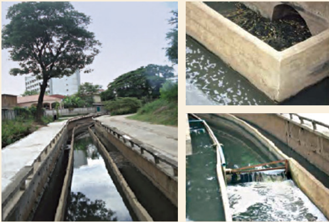
Water Diversion way in creek for divided wastewater and treated water
