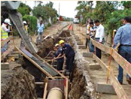
Construction of Sewerage System
