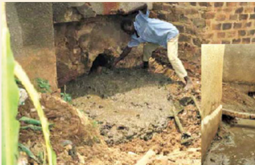
Manual pit emptying: unsafe and unhygienic
