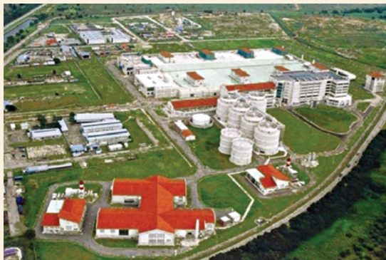
Changi Water Reclamation Plant
